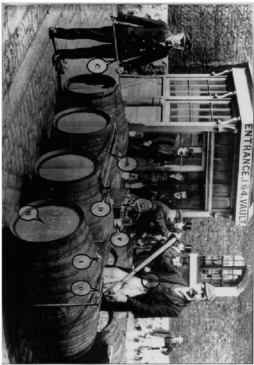
use of head and bung rods for measuring the diameters at the ends and bungs of the cask. He gives no description of these rods but notes that they are made by Mr John Gilbert, Mathematical Instrument Maker to the Custom House in London and the Out-Ports.
