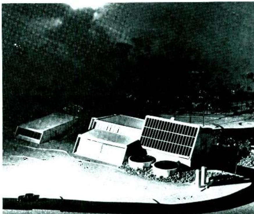
Fig. 1 — A highly energy-efficient wastewater treatment plant planned (by Wright, Pierce, Barnes and Wyman of Topsham, Me.) to use passive solar heating through large, all-south-facing windows, active solar collectors (dark panels), methane storage, heat pumps, etc.
