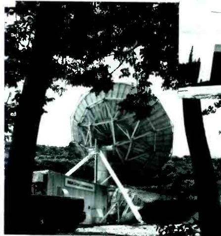
Fig. 2 — 33-foot earth station at Valley Forge.
